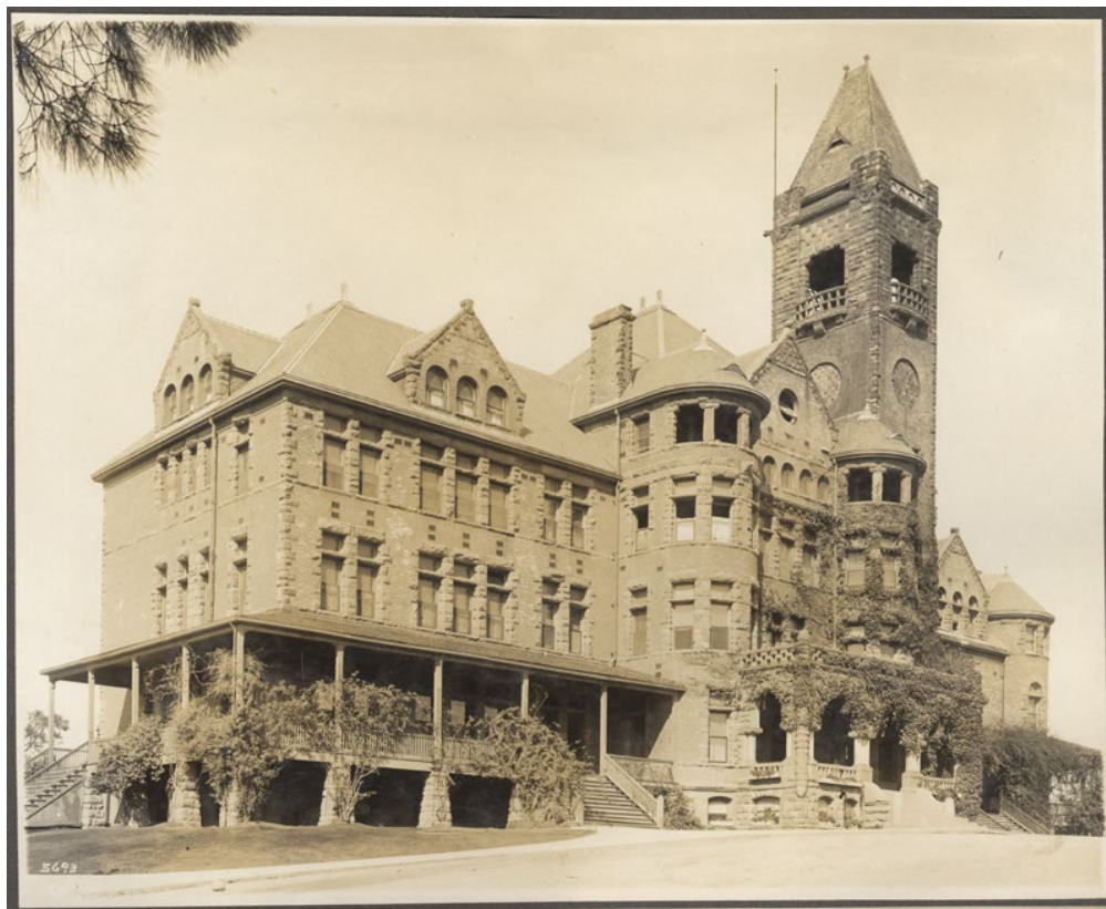
Figure 2. Administration Building “Preston Castle” at Preston School of Industry, ca. 1915 (McCurry Foto Co., California State Library, California Historic Section Picture Catalog, via Calisphere.org)
