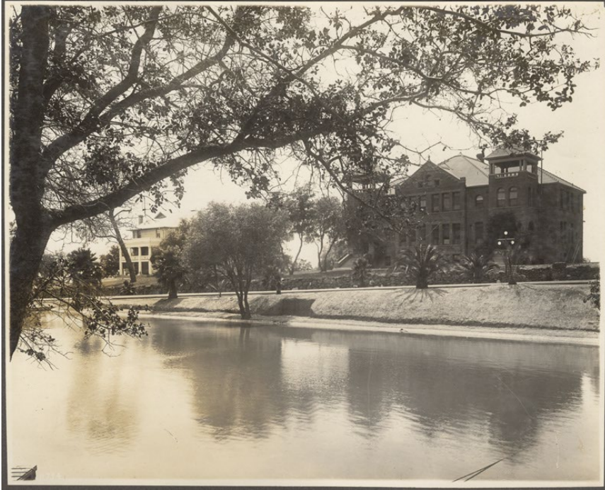
Figure 7. Grounds at Preston School of Industry with swimming pool in foreground, Honor College No. 1 “The Colonial” at left-background, and West Cottage right-background (McCurry Foto Co., California State Library, California Historic Section Picture Catalog, via Calisphere.org)
