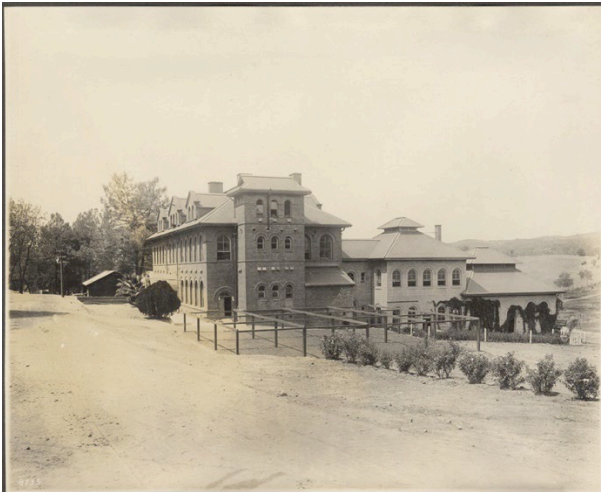
Figure 5. The Romanesque Revival style Trades Building, designed by architect Henry A. Schulze, ca. 1915 following its refurbishment and the addition of shops at its rear ca. 1908 (McCurry Foto Co., California State Library, California Historic Section Picture Catalog, via Calisphere.org)
